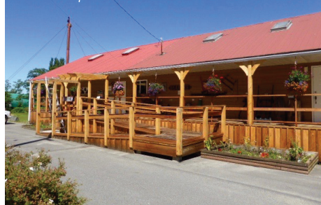
New ramp at the Port Clements Museum
